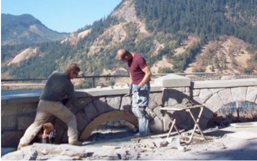
Stone masons Rick Olmstead and Josh Maiden work last month on the Mitchell Point State Park overlook. Rick is the son of Don Olmstead, owner of Nature's Edge Stone Art Inc., one of a small number of companies that can meet federal criteria for matching historic stone walls in repair and expansion projects.
